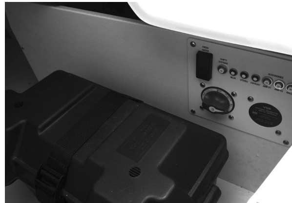
Figure J2: Fresh Water Switch on Battery Switch Panel (Locations May Vary Depending on Model)
