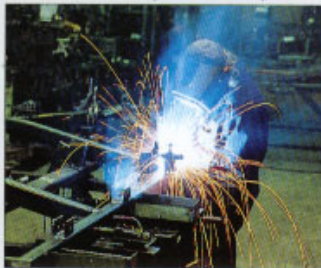
Welder Dave Smith follows rigid quality control standards at the Four Winns Trailer Plant.
