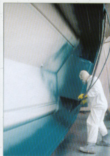
Jim Crain applies 25 mils of Armorcote.
