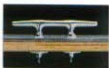
Cleats are through-bolled and metal-backed.
